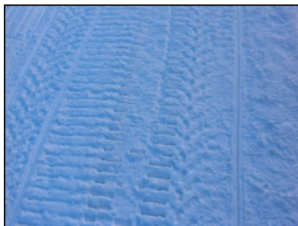
Photo 108: Surface chew and skag marks from slow pass-by
